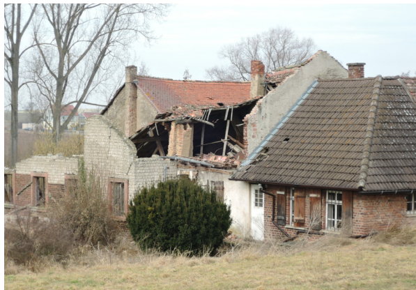
Active reuse instead of landfilling
